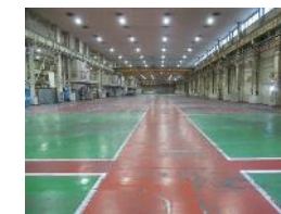
September: Large crane installed Preparation of BSF organization structure completed
